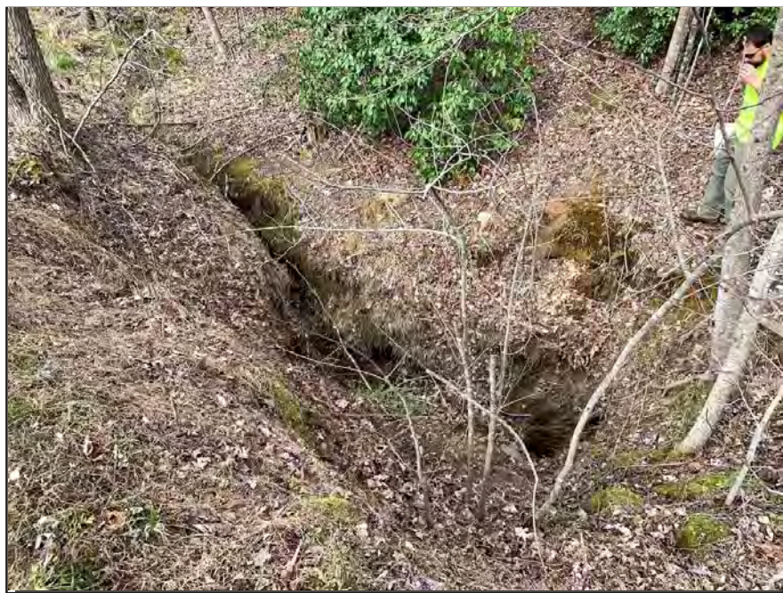
Photograph 20: Downstream Face, 2020 – heavy vegetative growth surrounding drainage channel from the downstream face.
