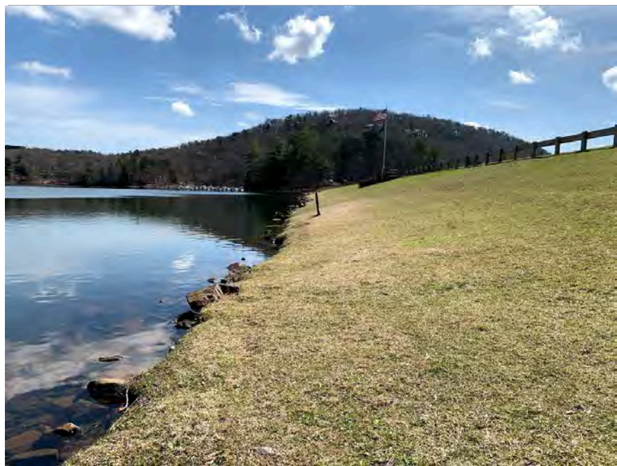
Photograph 2: Upstream Face, 2020 – localized areas of erosion and beaching along shoreline.
