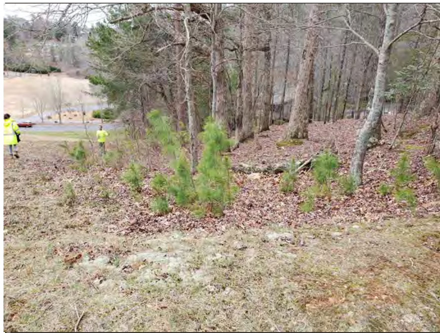
Photograph 14: Downstream Face, 2020 – vegetation along the right and left abutments have begun encroaching on the groin, slopes, and benches again.
