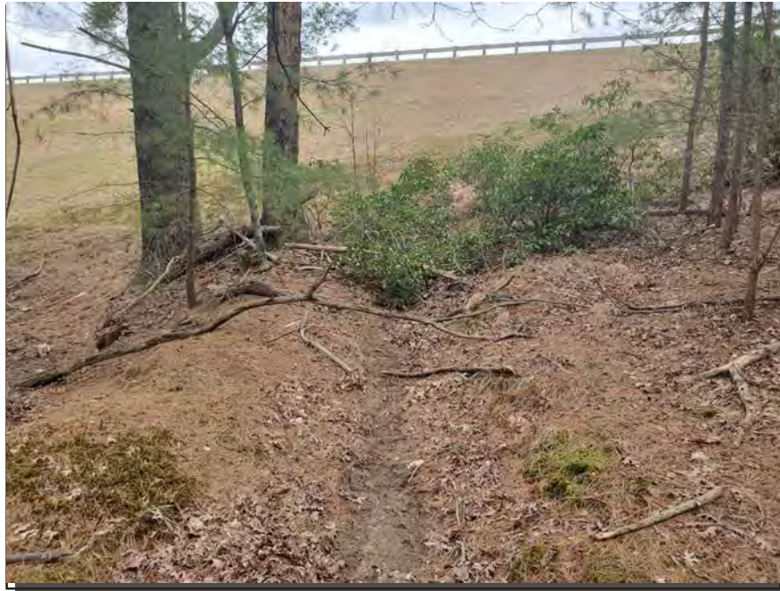
Photograph 13: Downstream Face, 2020 – debris at the abutment of a bench that could obstruct the path of stormwater flow and lead to surficial erosion on the slope downstream.
