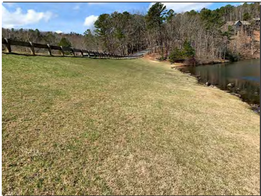
Photograph 4: Upstream Face, 2020 – slope surface with no erosion midway up the western half of upstream face.
