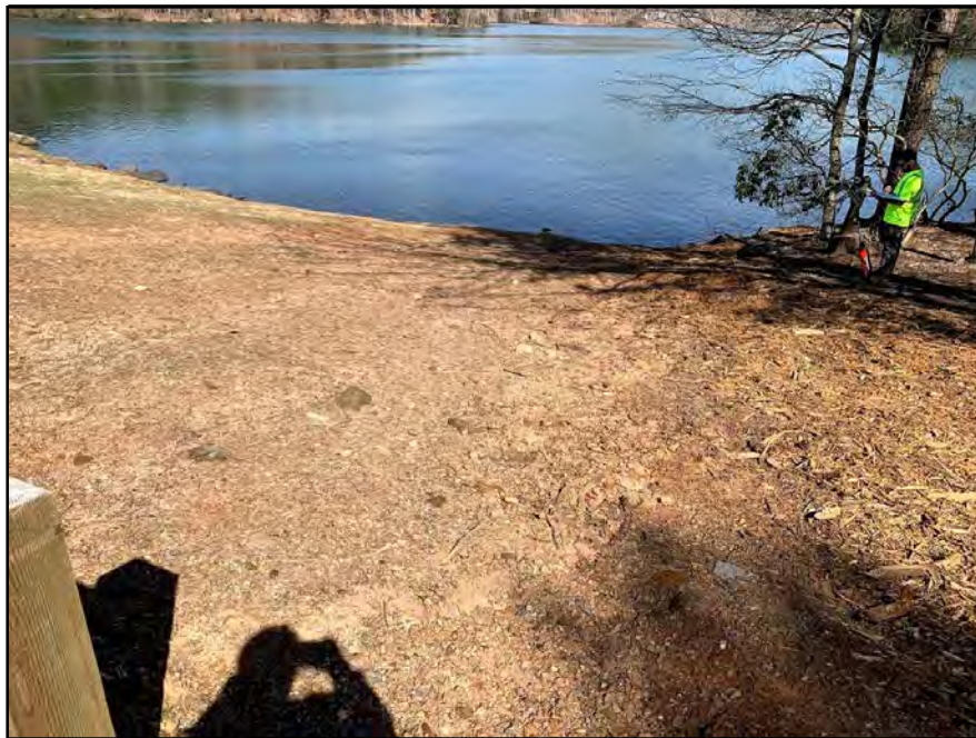
Photograph 9: Upstream Face, 2020 – erosion at left groin from foot traffic and surface water runoff.
