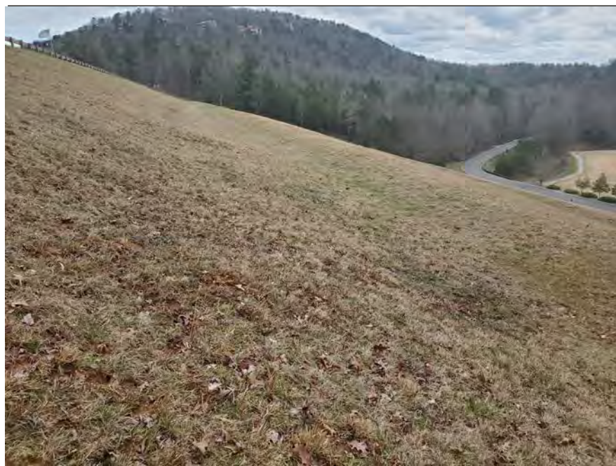
Photograph 10: Downstream Face, 2020 – general conditions as viewed from right abutment.
