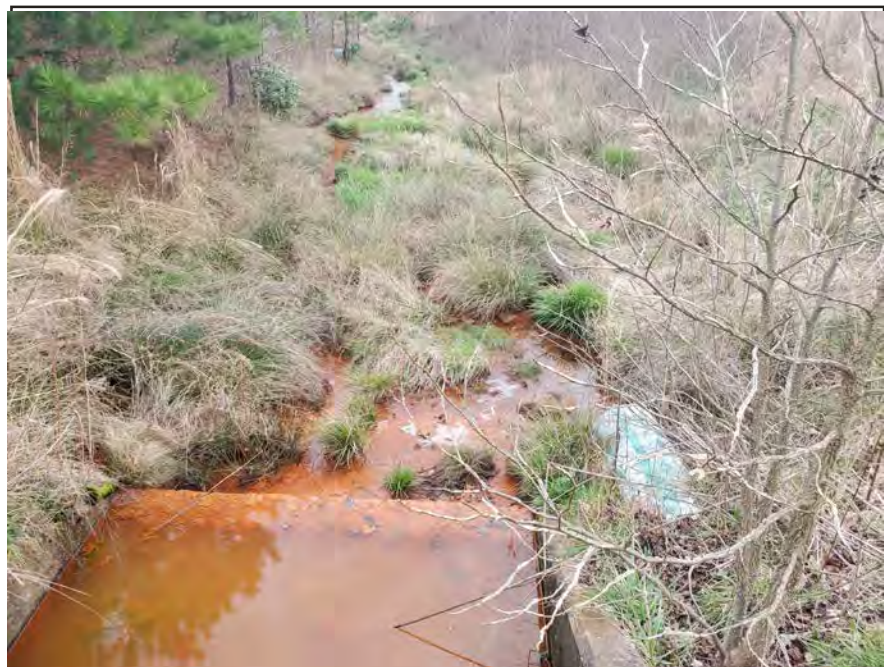
Photograph 22: Tail Water Creek, 2020 – view of the low-level outlet concrete stilling basin discharge to the tailwater creek.
