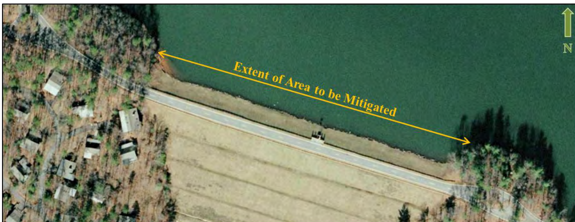
Figure 1: Lake Petit Dam extent of area where minor “beaching” erosion has been observed and is to be mitigated.
